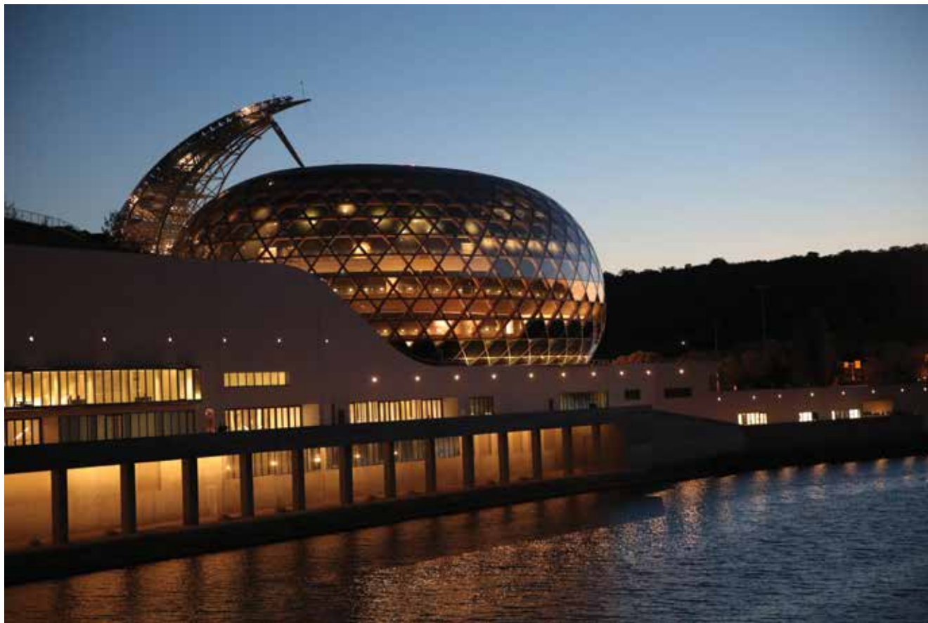
La Seine Musicale, complex of buildings on the island opened in April 2017, located between Boulogne- Billancourt and Sèvres, in the western suburbs of Paris, on the Seine. A large sail-like curved solar panel provides most of the site's daytime energy needs.
